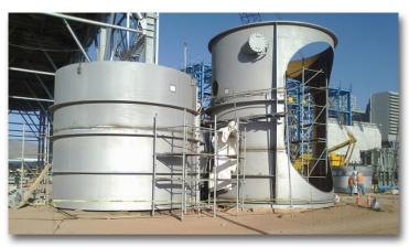
Supply, Fabrication and Painting of Exhaust Steam Duct, Steam Distribution Ducts, Condensate Tank and Drain Pot.
